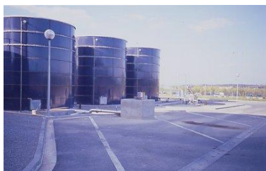
Picture E.1: Reception Tanks
