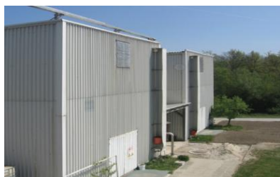
Picture F.4: Biogas tank
