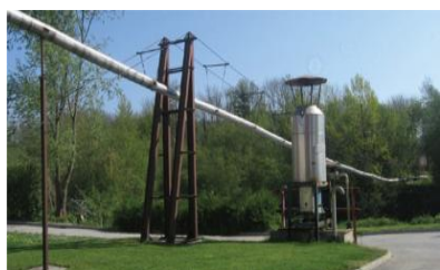
Picture F.1: Reception pig manure pipe
