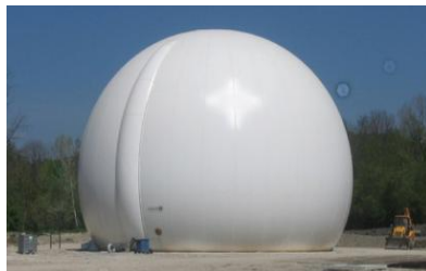
Picture F.5: Biogas balloon
