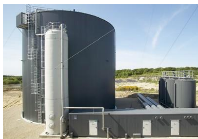
Picture A.2: Anaerobic digester (reactor, 7,000 m 3 ).
