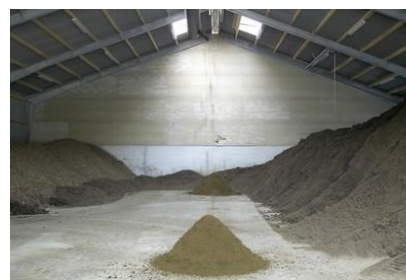
Picture A.4: Storage facility for solid fraction.
