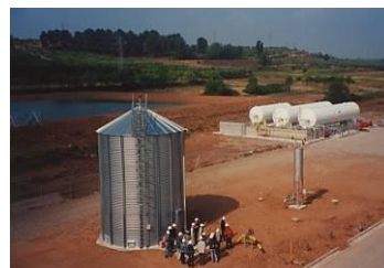
Picture E.3: Gas holder and flare
