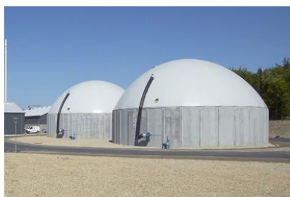
Picture A.3: Gas storage.
