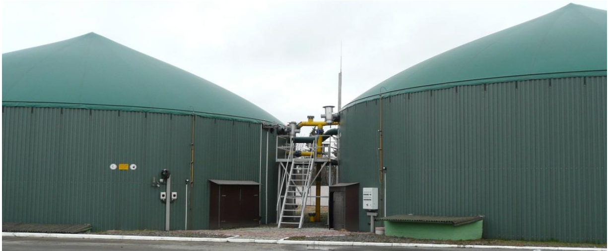
Picture 5: Biogas Plant “Belorusky”. Between two digesters the yellow pipe grants for the overflow of biomass (source: Kuzina)
