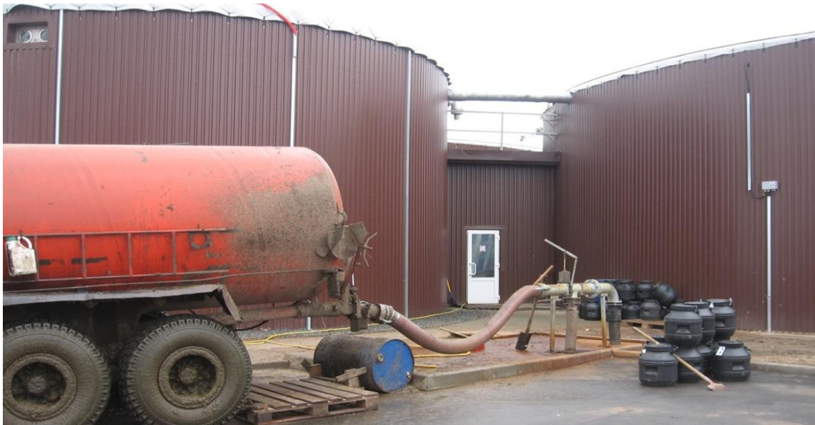
Picture 5: Pumping of liquid biomass into the digester from a slurry tanker on the biogas plant at the “Snov” farm (source: Kapustin)
