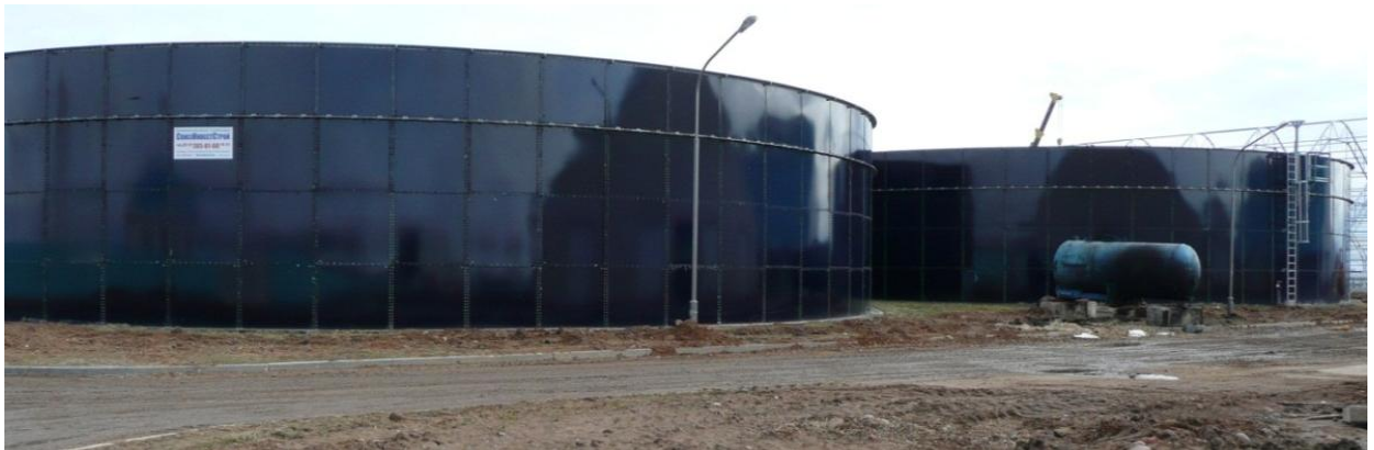
Picture 3: Primary and secondary digesters of biogas Plant “Zazerye” the 28.03.2012 (source: Kuzina)
