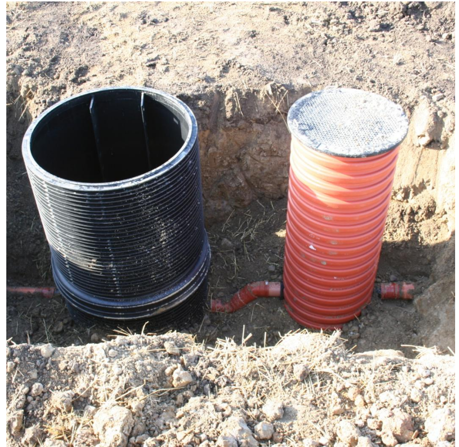
A WELL FOR MEASURING WATER FLOW (LEFT) AND A REGULATION WELL FOR CONTROLLED DRAINAGE BEING INSTALLED AT HOFMANSGAVE.
