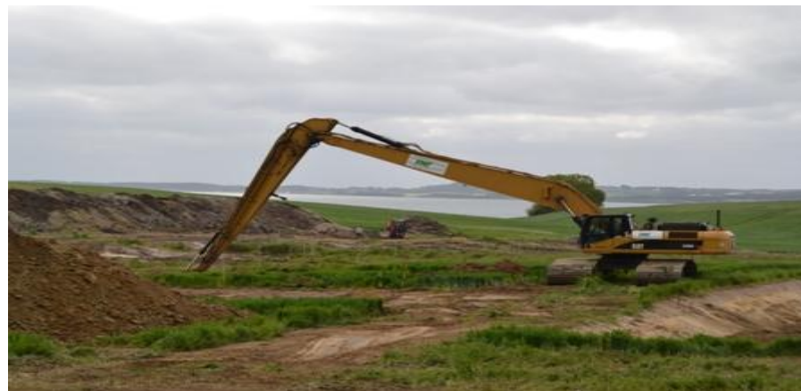
DIGGING OF RESERVOIRS FOR CULTIVATION OF ALGAE IN DRAINAGE WATER (FROM HTTP://2.NATURERHVERV.FVM.DK ).
