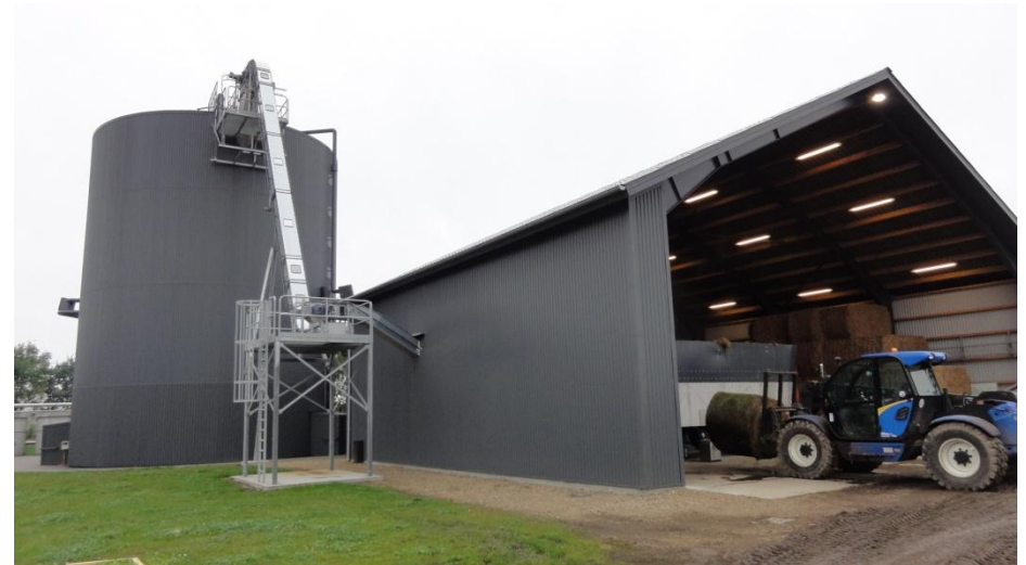
AT AU FOULUM'S BIOGAS PLANT ROUND BALES OF WILTED MEADOW GRASS IS LOADED INTO THE BIO-MIXER, WHICH AFTERWARDS FEEDS IT TO THE EXTRUDER, FROM WHERE IT IS FED INTO THE DIGESTER TANK. BESIDES FROM THE LOADING, THE PROCESS IS REGULATED AUTOMATICALLY.
