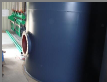
Lower part of the settling tank.
