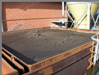
Sludge bed of the pilot installation, with cover/lid removed.
