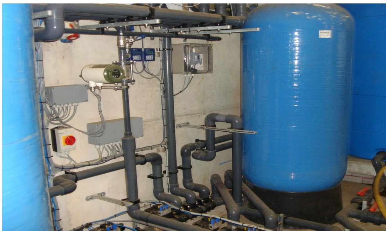
Picture 9: The liquid fraction is de-mineralised in the final step before being deposited in the nature.
